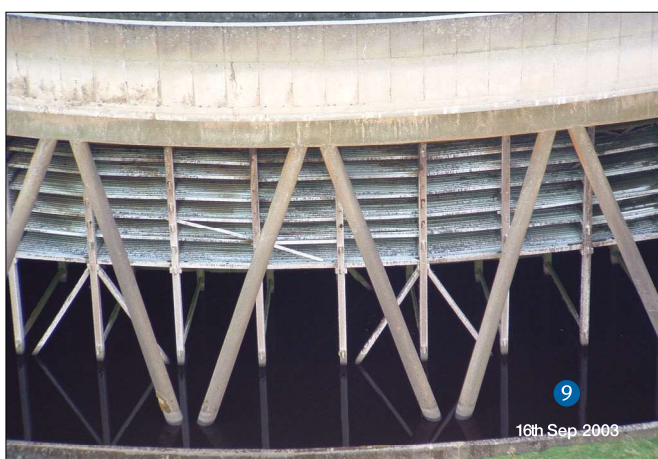
5. Interior View of Generating Hall. 6. Cooling Tower Structural Detail. 7. Detail of Extract Chimneys and Conveyor Belt. 8. Peat Wagon Tipper. 9. Base of Cooling Tower.
