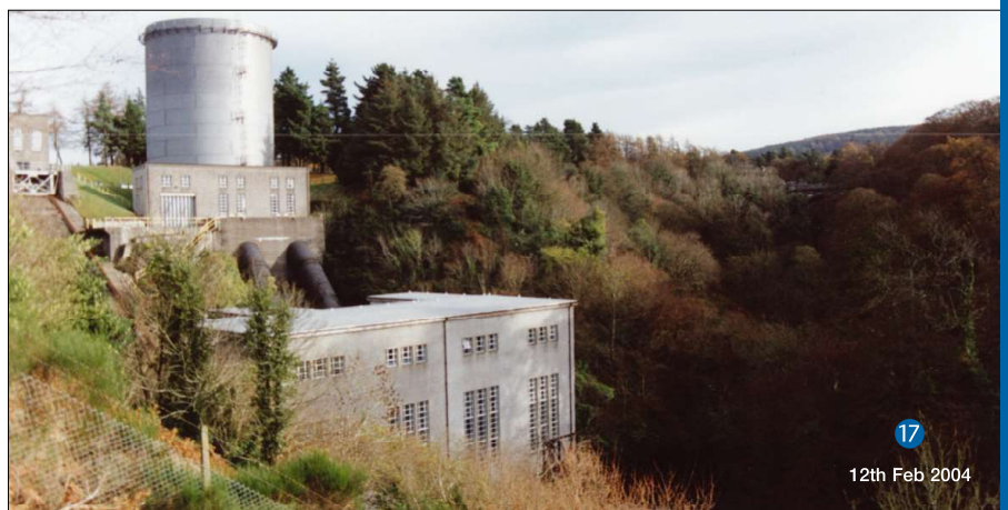
14. Detail of Dam Spillway Gates. 15. Oblique View of Dam. 16. Detail of Dam Intake House. 17. Elevated view of Complex.
