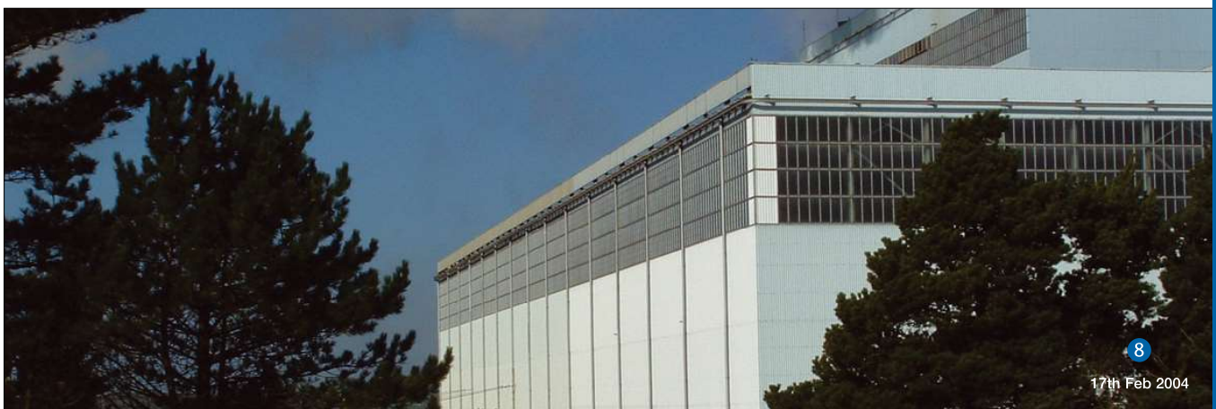
5. View of Complex looking North towards Co. Clare. 6. Turbine Unit No. 4. 7. Turbine Units No. 1 & 2. 8. External View of Generating Hall.
