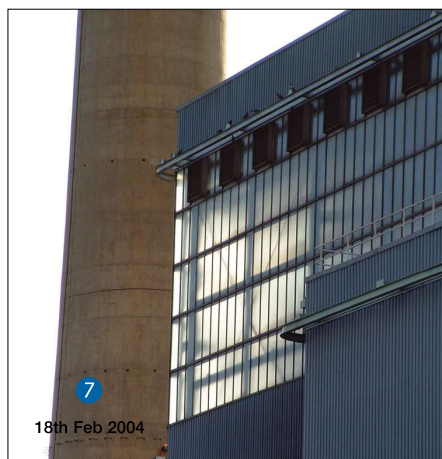
4. View of Complex from Jetty. 5. Cooling Water Busmain adjacent to Cooling Water Pump House. 6. Interior of Cooling Water Pump House. 7. Detail of Power Station Clerestory Fenestration.
