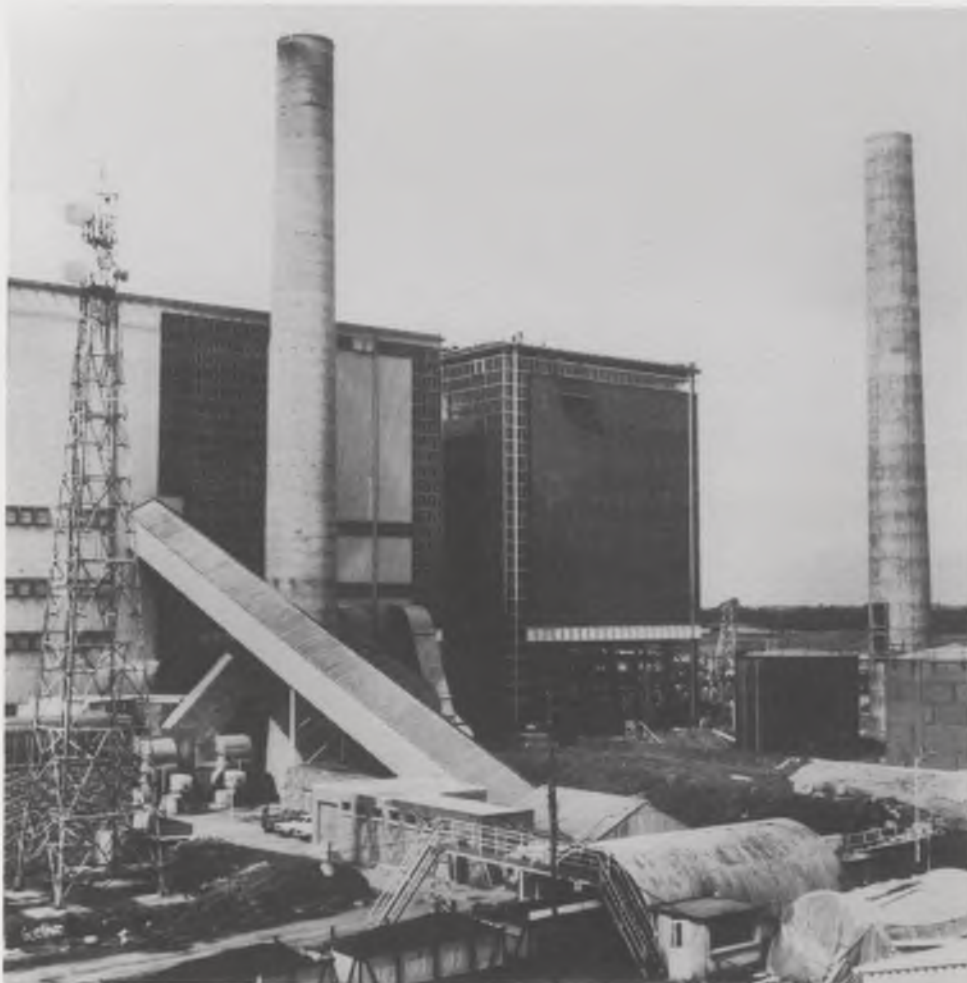
View of Fuel Handling Plant
