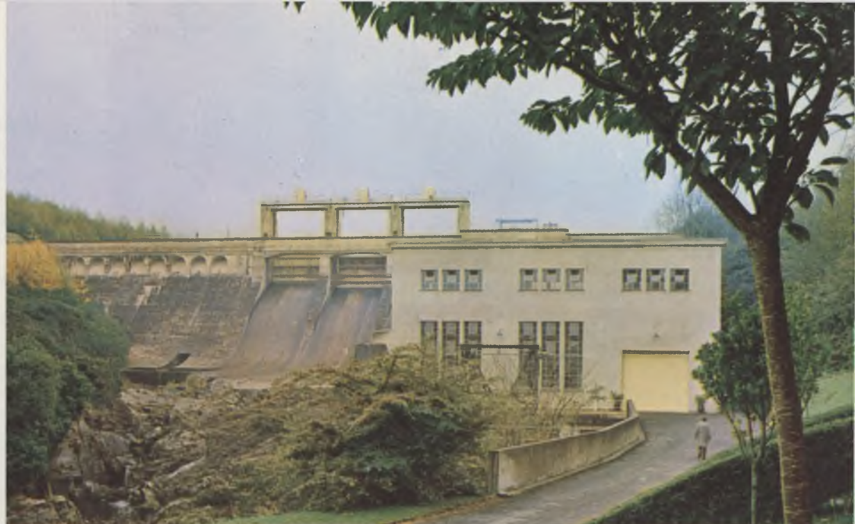
Above: Golden Falls Generating Station
