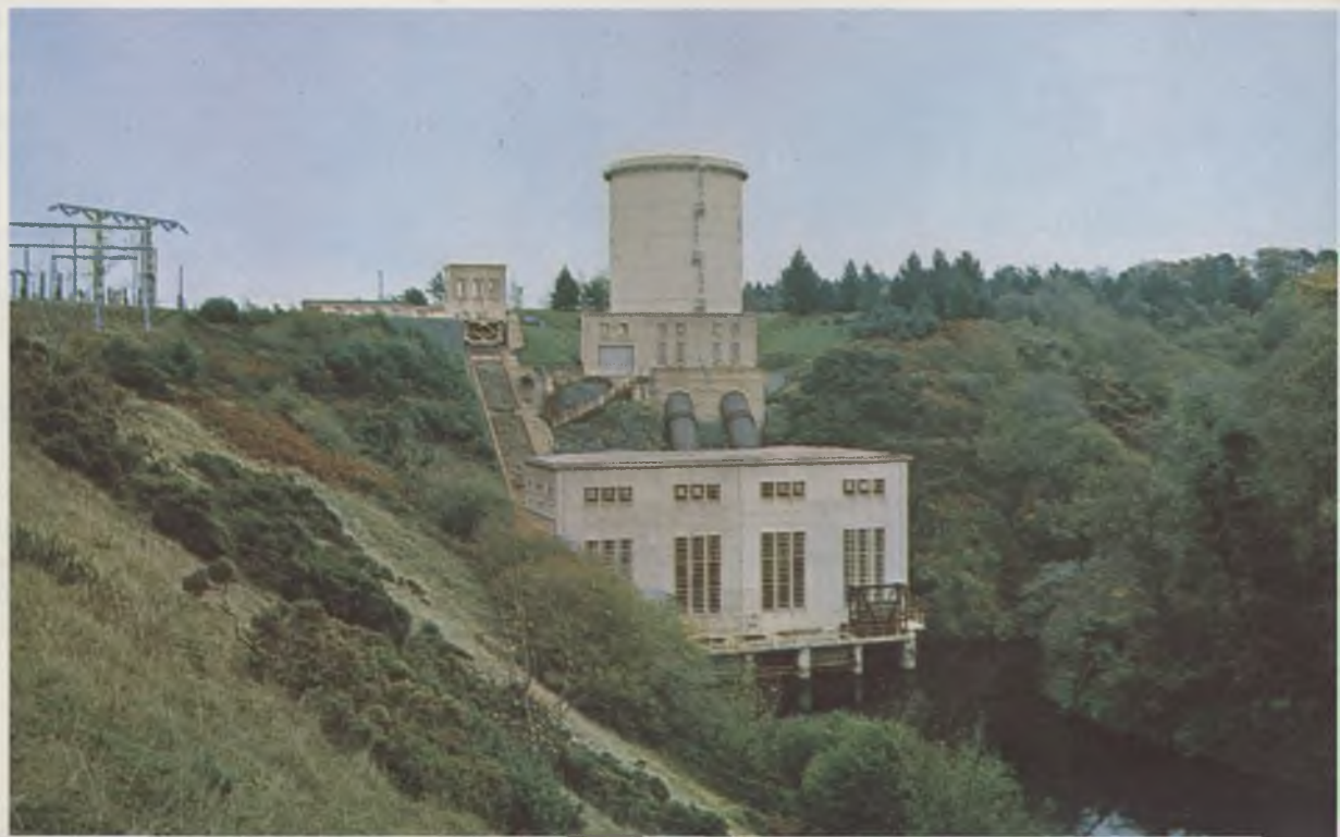
Below: Pollaphuca Generating Station
