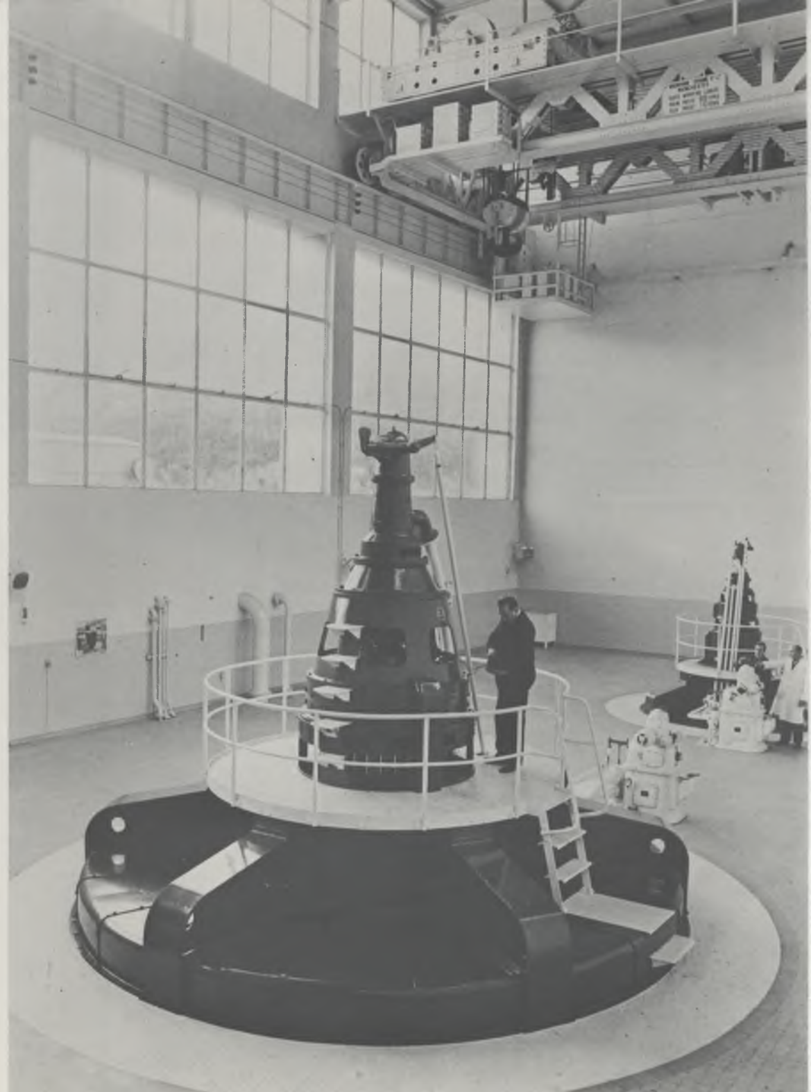
The Generating Hall, Inniscarra
