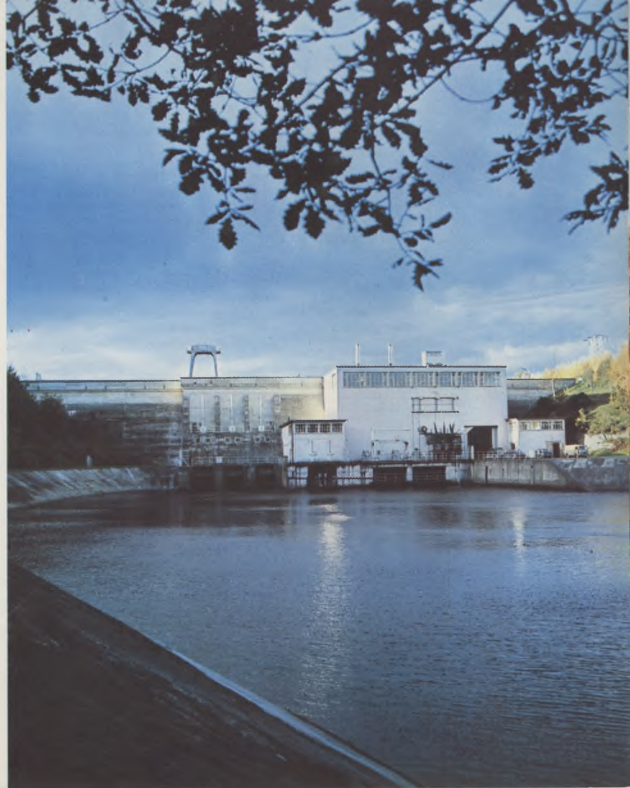
Carrigadrohid Generating Station
