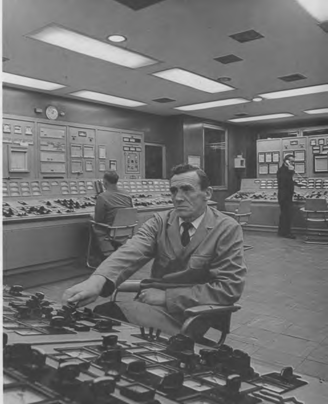
Thermal Control Room
