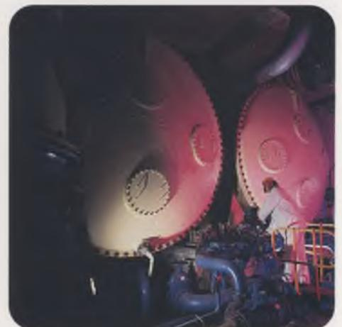
the gas turbine still retain sufficient energy to produce high pressure and temperature superheated steam in a Heat Recovery Boiler. This steam is then directed to a Siemens Turbo-Generator where a further 30 MW's of power is produced.
