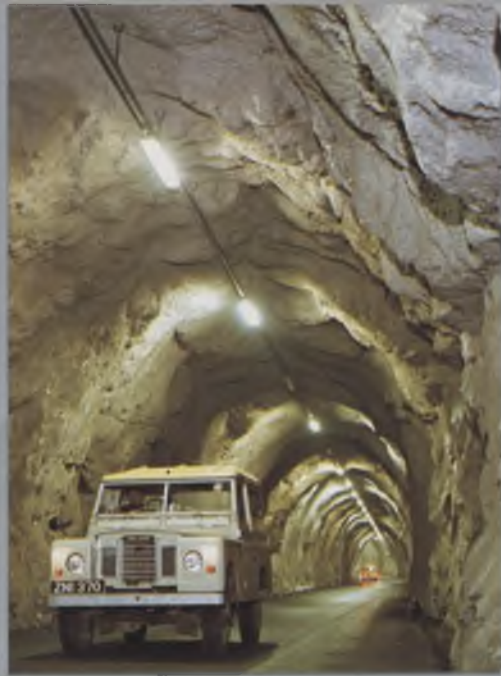
The access tunnel leading to the main cavern.
