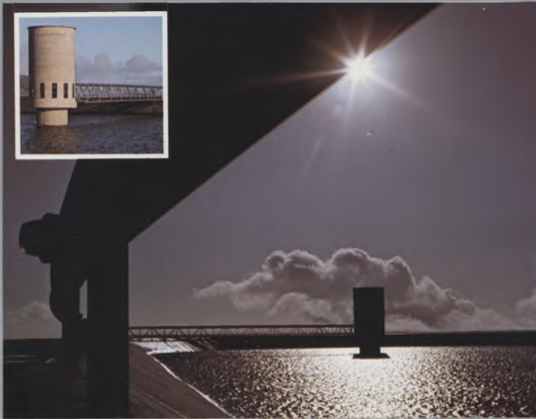
The completed upper reservoir. Inset shows intake structure.
