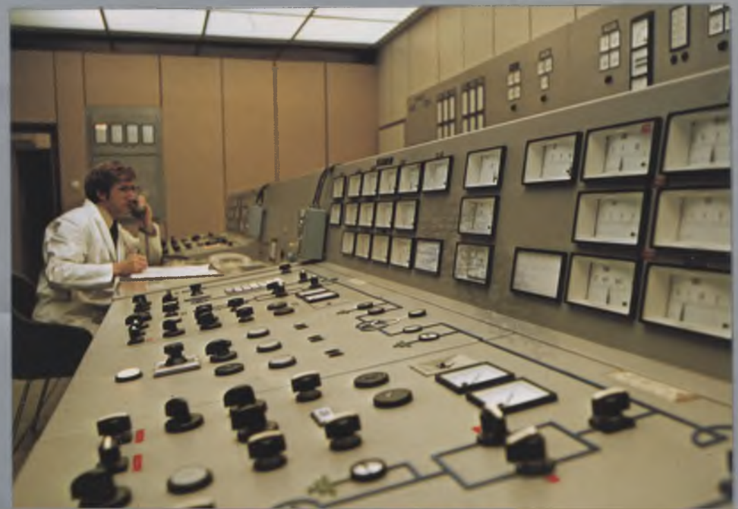
The control room.
