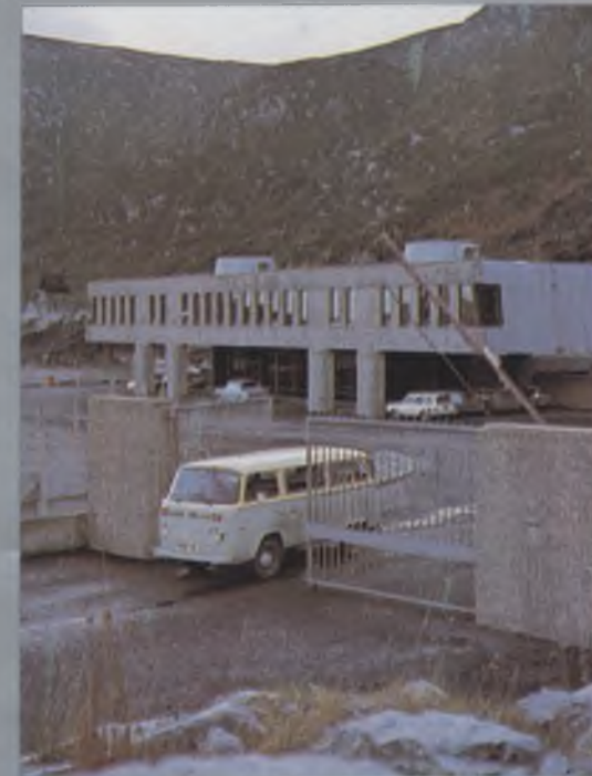
The administration building.
