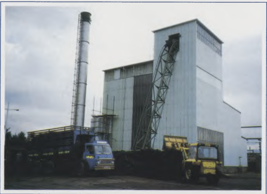
Unloading and bunkering
